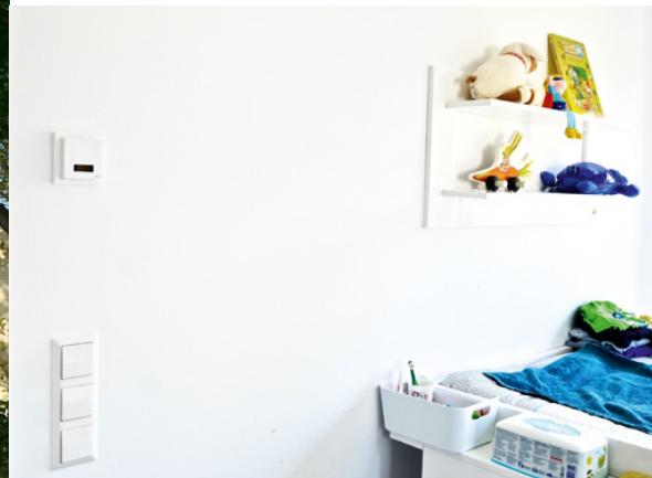
The maintenance-free Eltako FTF65S temperature sensor is supplied from the integrated solar cell with energy store.
