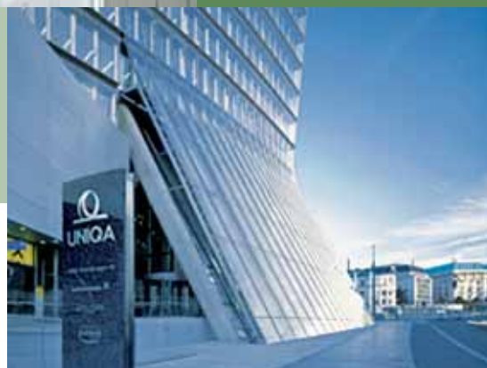
UNIQA company head offices in Vienna: 500 EnOcean radio-based room sensors on 22 floors
