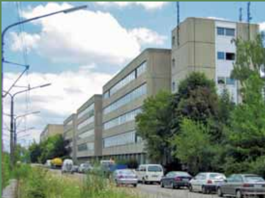
Siemens Munich: light and blinds control in 11 office buildings using EnOcean radio sensors
